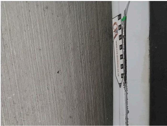
9: Sill os Dented With Paint Damage
